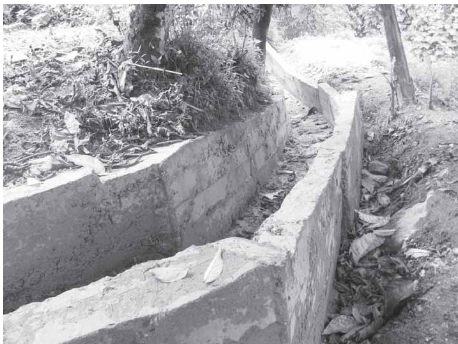
Box Drain built under NREGS in Kabi
