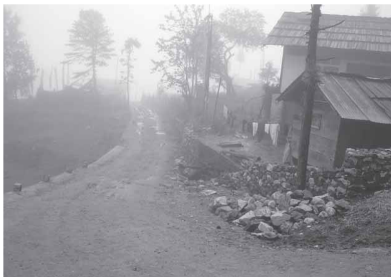
Jeepable road constructed under NREGS in Lachung, North District
