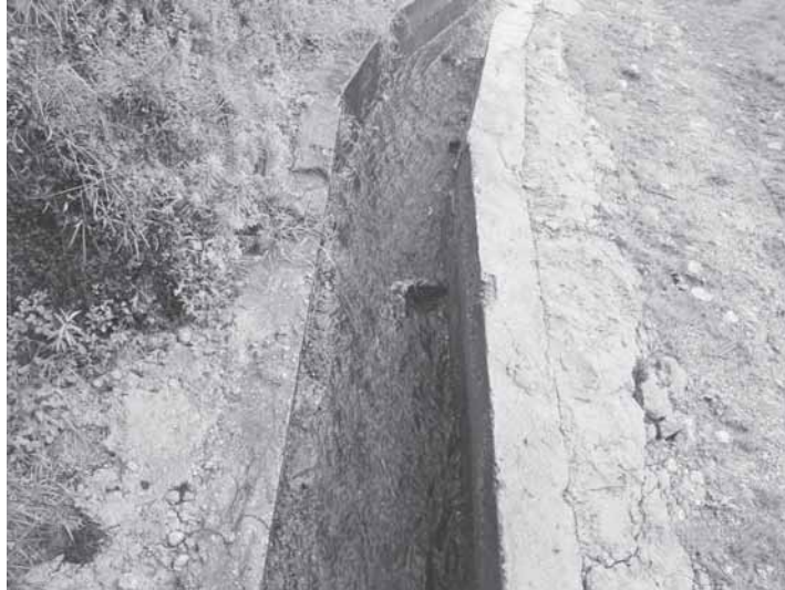
Box Drain built under NREGS in Kabi
